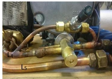
Figure 3. Manual valve (upper) and thermostatic valve (lower) in parallel. Connection lines L<sub>4</sub> and L<sub>5</sub>.
