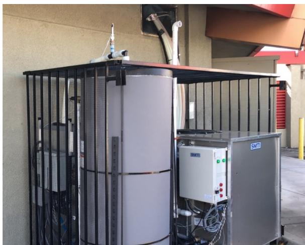
Figure 1: Commercial Gas Heat Pump Skid Package Installed at Host Site
